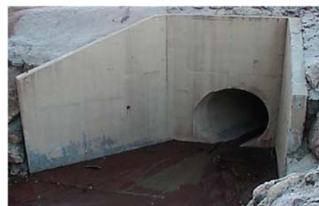
Fig.2. schematic of wingwalls and headwall
