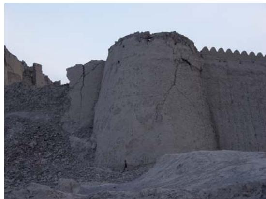
Fig. 2 - Damages to tower No. 32 and its eastern wall
