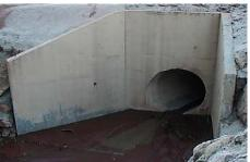
Fig.2. schematic of wingwalls and headwall
