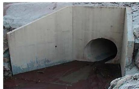
Fig.2. schematic of wingwalls and headwall
